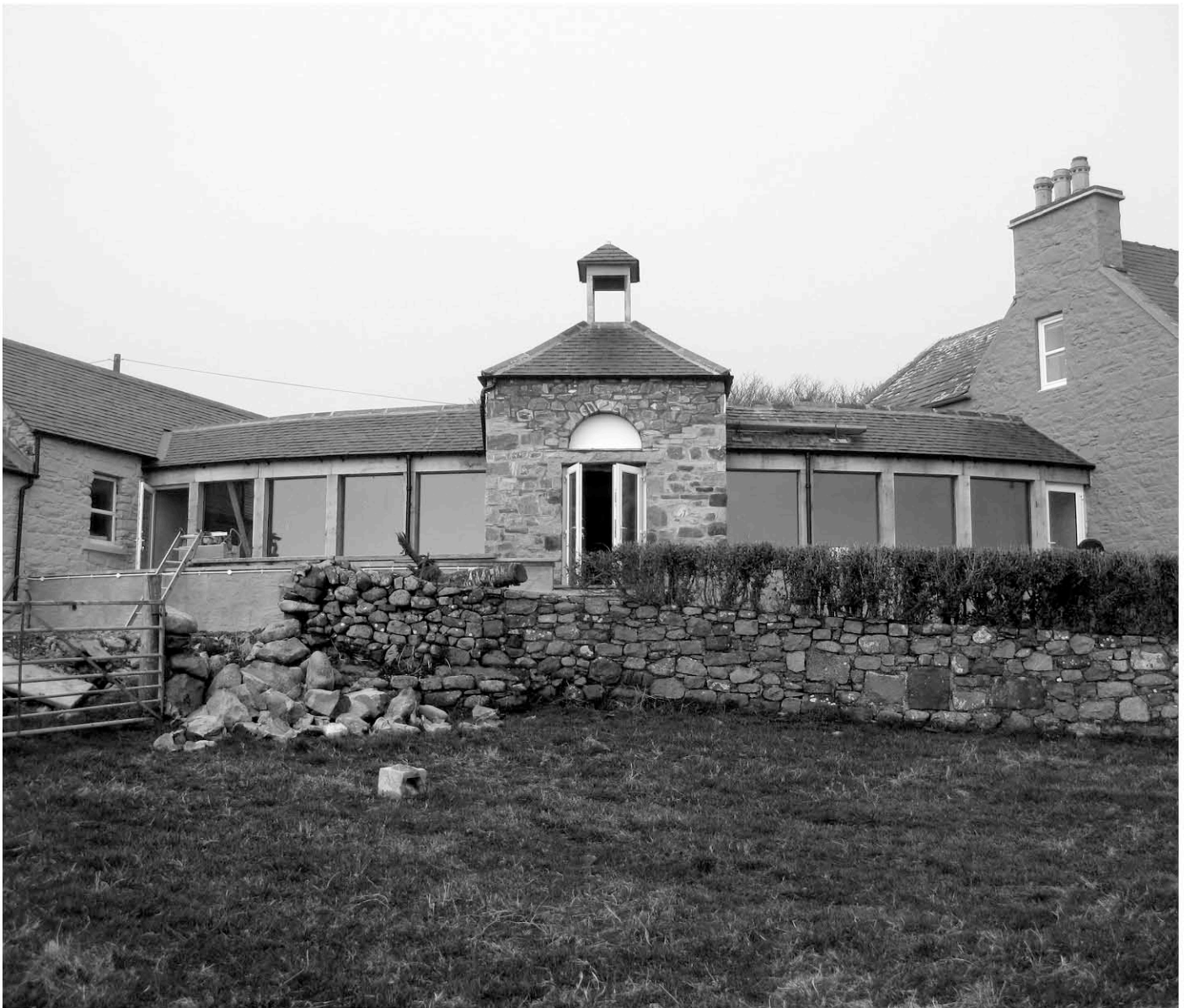
Links pavilion nearing completion.
